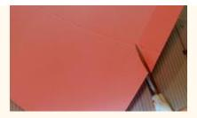
At the 11" score line, cut at an angle from the edge up to the score line, removing the excess and creating a tab.
